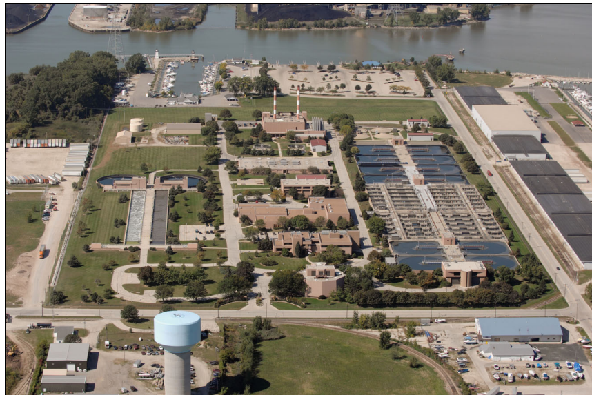
GBMSD Green Bay Facility at the Mouth of the Fox River
