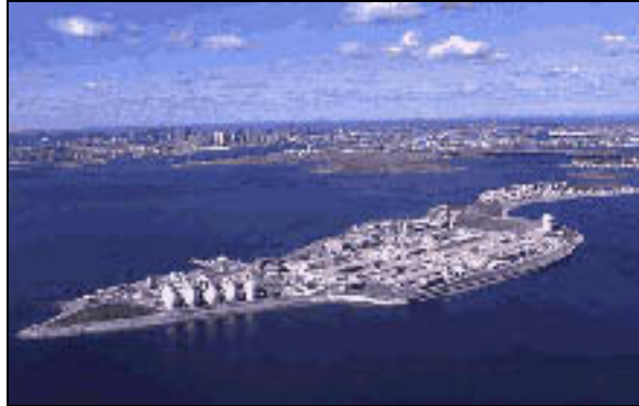
MWRA Deer Island Wastewater Treatment Plant
